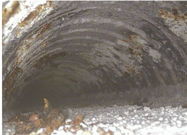
Figure 8.10. Bore scope picture looking toward highpoint in tendon 1
