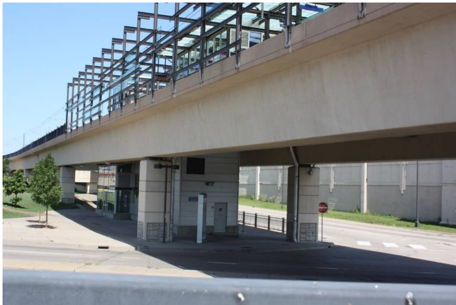
Figure 5.1. Overview of bridge 27262
