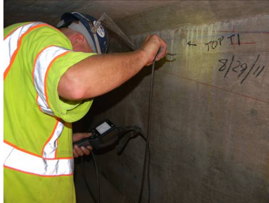
Figure 3.3. Use of borescope into post-tensioning duct
