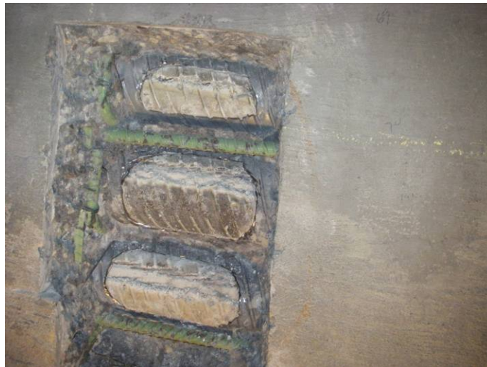
Figure 8.6. Exposed ducts in girder 5 of span 2
