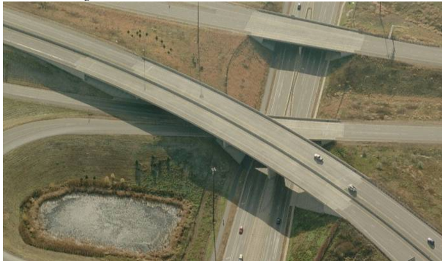
Figure 4.8. Bridge 02037 E aerial view (Bing, 2011)
