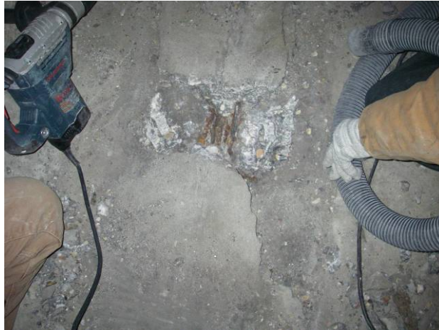
Figure 6.31. Removal of concrete exposing tendon B28
