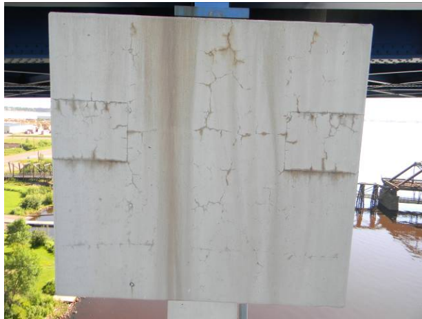
Figure 9.1. PT cap on Blatnick Bridge pier
