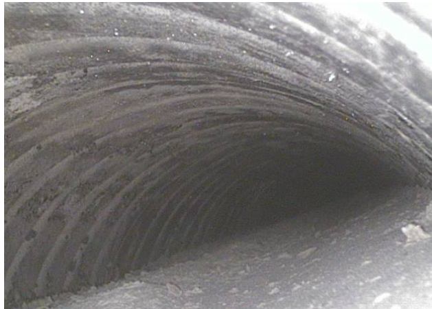
Figure 8.13. Boreoscope picture looking toward low point in tendon 2
