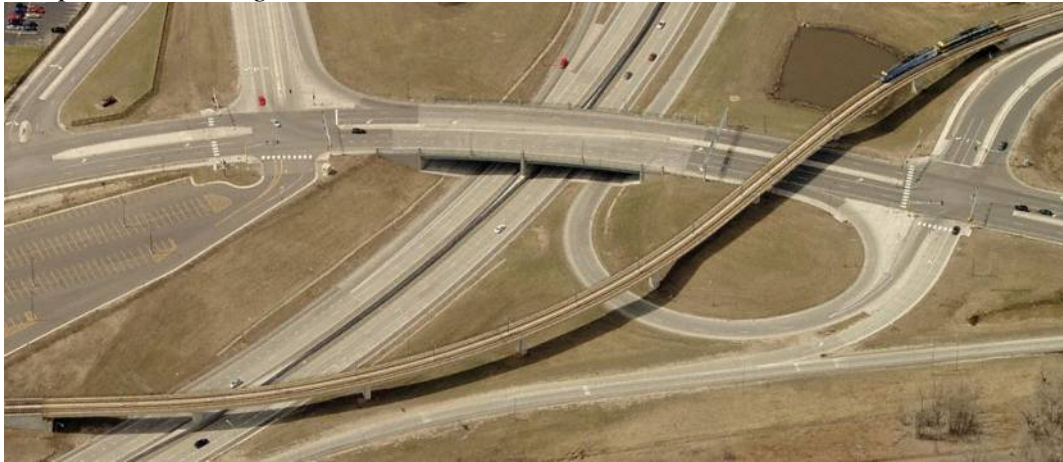
Figure 4.5. Bridge 27262 aerial view (Bing, 2011)
