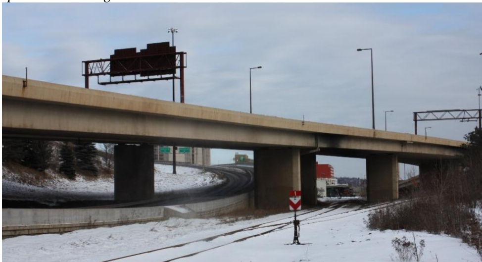
Figure 4.18. Bridge 69818 N ground view
