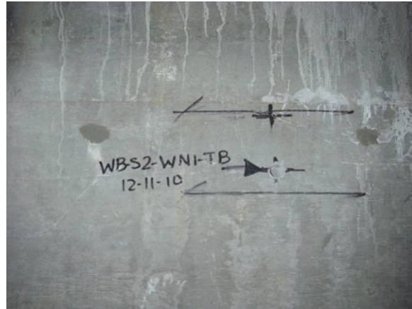
Figure 6.14. Overview photo of drilled hole into span 2 web S2 tendon B
