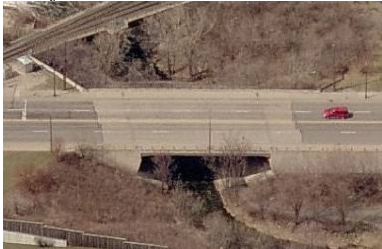
Figure 4.15. Bridge 27719 aerial view (Bing, 2011)
