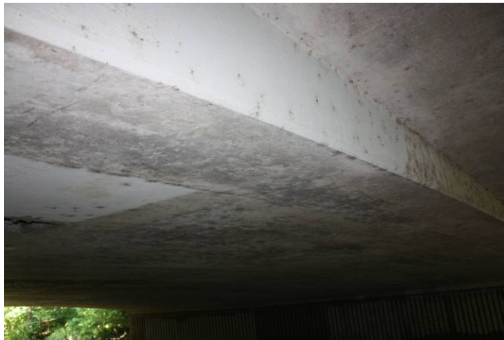
Figure 5.13. Slab span of bridge 27547
