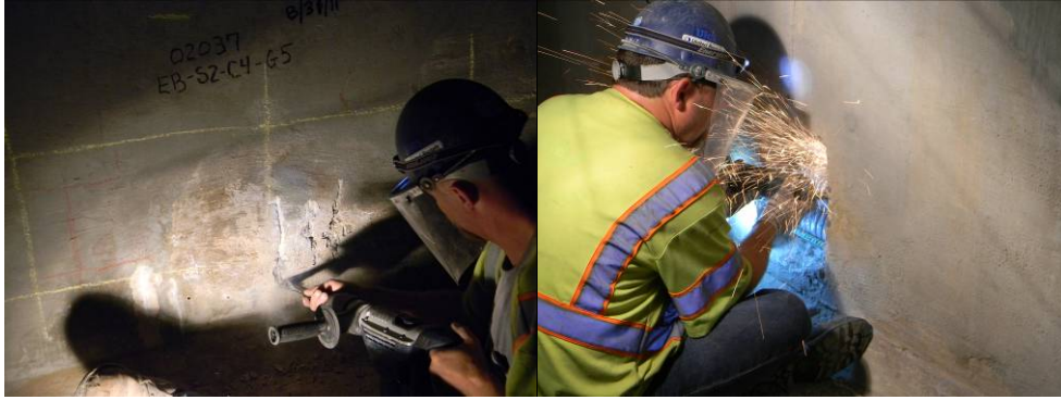
Figure 3.6. (Left) Exposing post-tensioning duct by cutting web
