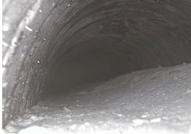
Figure 8.12. Boreoscope picture looking toward highpoint in tendon 2
