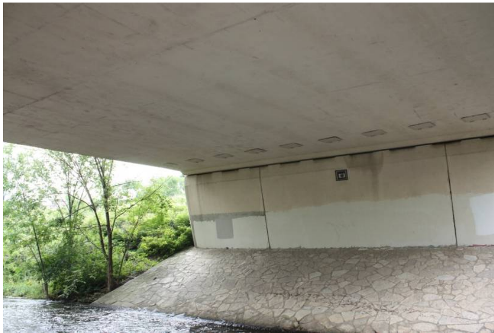
Figure 5.7. Bridge 27719 overview picture
