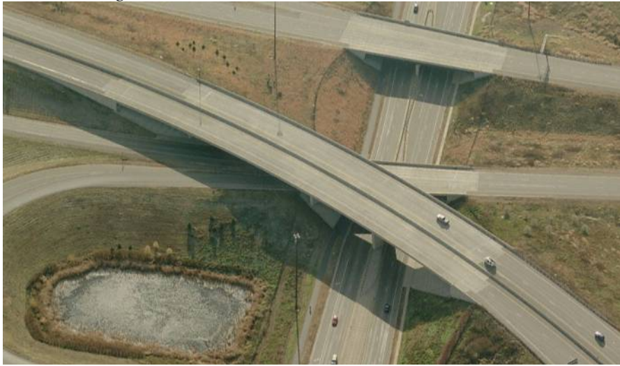
Figure 4.11. Bridge 02037 W aerial view (Bing, 2011)
