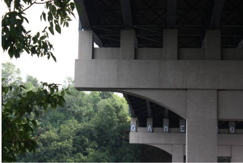
Figure 5.5. Main spans across the Mississippi River
