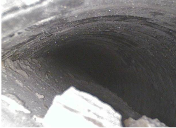
Figure 8.14. Borescope picture looking toward highpoint in tendon 3
