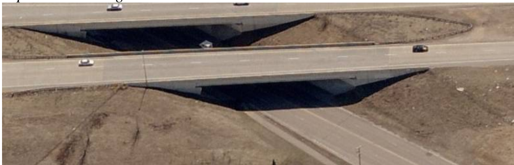
Figure 4.39. Bridge 70038 aerial view (Bing, 2011)
