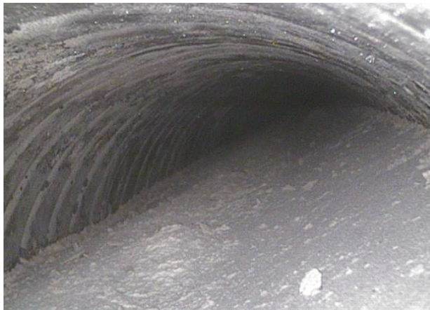
Figure 8.15. Borescope picture looking toward low point in tendon 3
