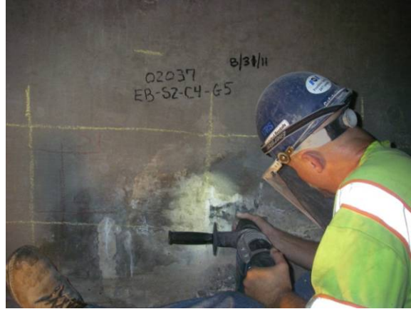
Figure 8.5. Removing cover at inspection area
