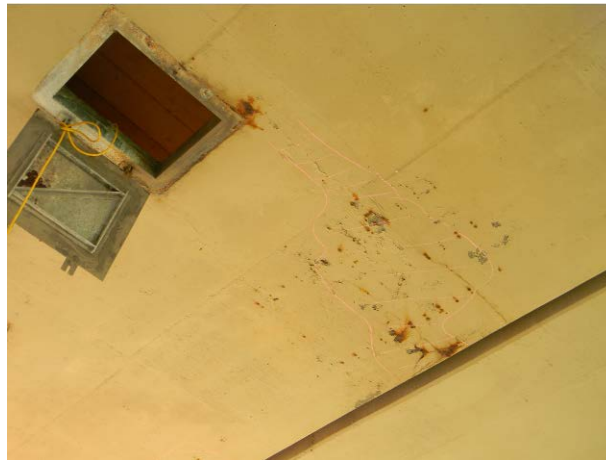
Figure 7.9. Access hatch for structural unit 6N
