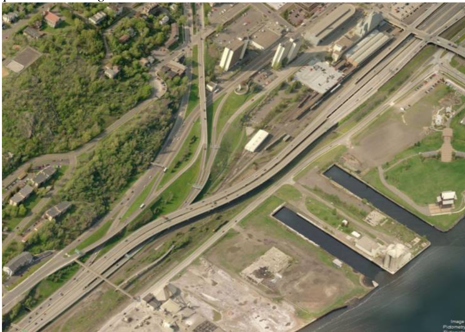
Figure 4.28. Bridge 69818 S aerial view (Bing, 2011)
