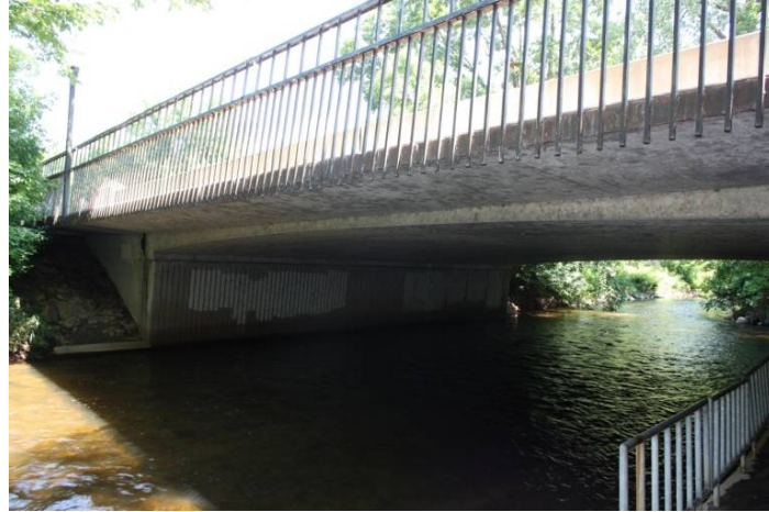
Figure 5.12. Bridge 27547 spanning across the Minnehaha Creek
