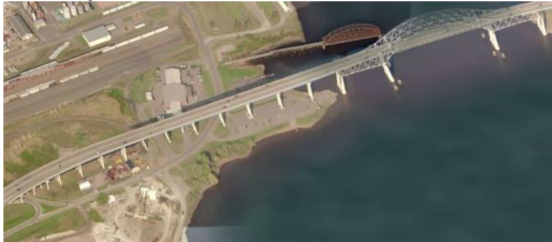
Figure 4.33. Bridge 9030 aerial view (Bing, 2011)
