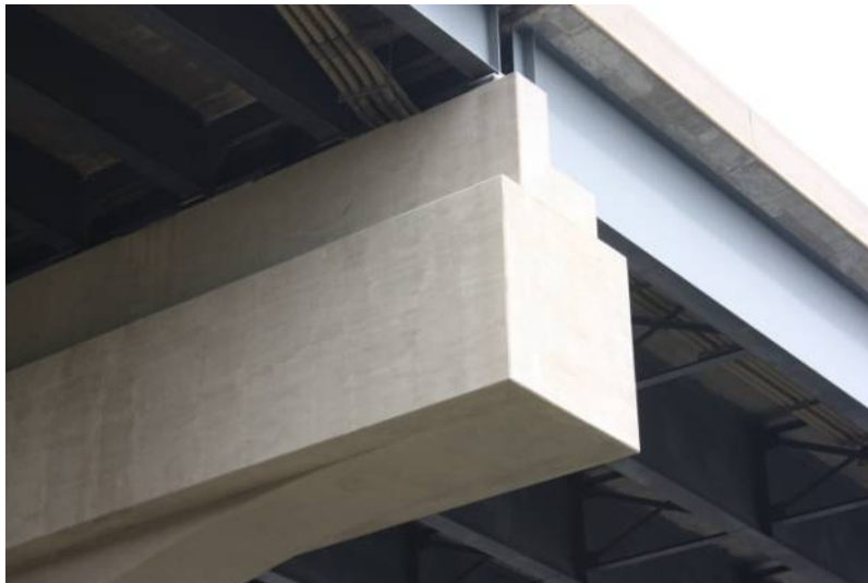
Figure 5.6. Post-tensioned pier cap
