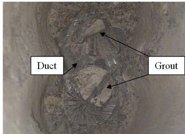
Figure 8.9. Boreoscope picture of drilled hole in girder 5 of span 2
