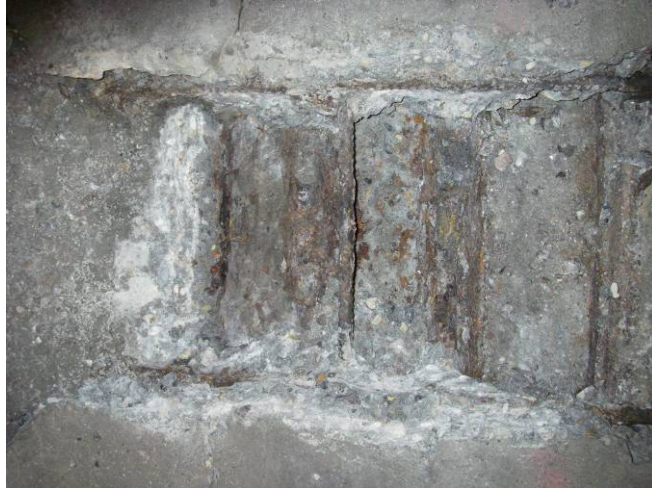
Figure 6.23. Overall view of opened/chipped area at mid span
