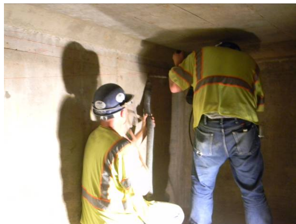
Figure 3.2. Drilling into post-tensioning duct
