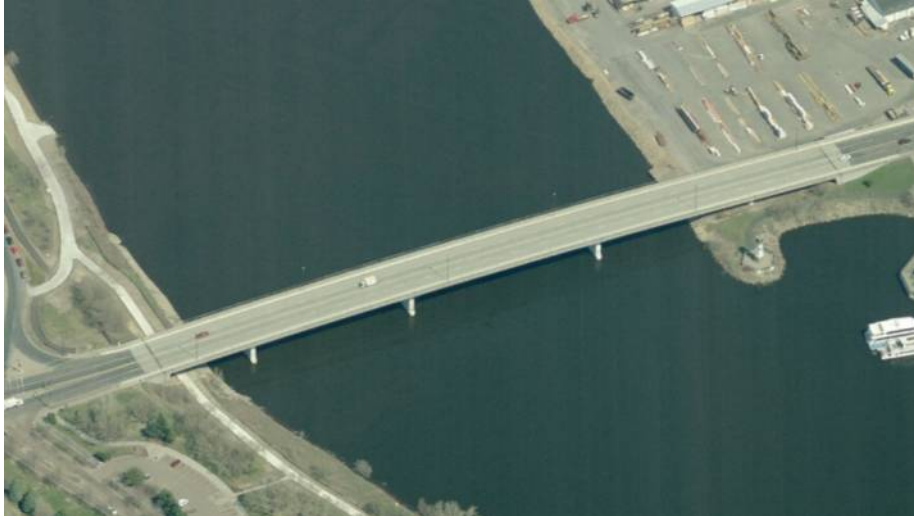
Figure 4.1. Bridge 27611 aerial view (Bing, 2011)
