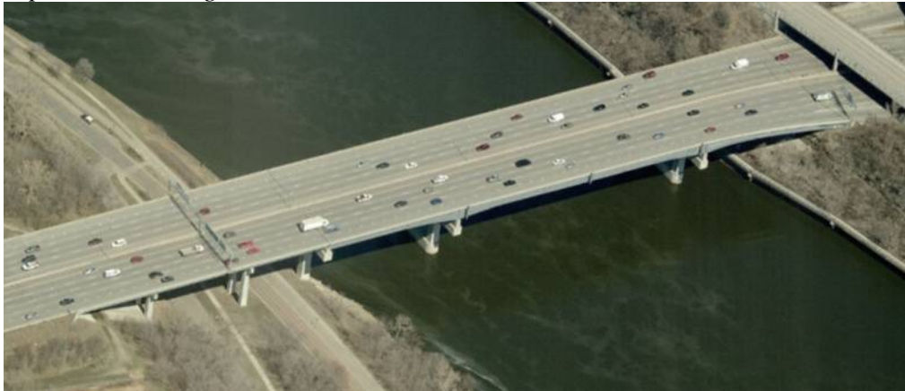
Figure 4.14. Bridge 9350 aerial view (Bing, 2011)
