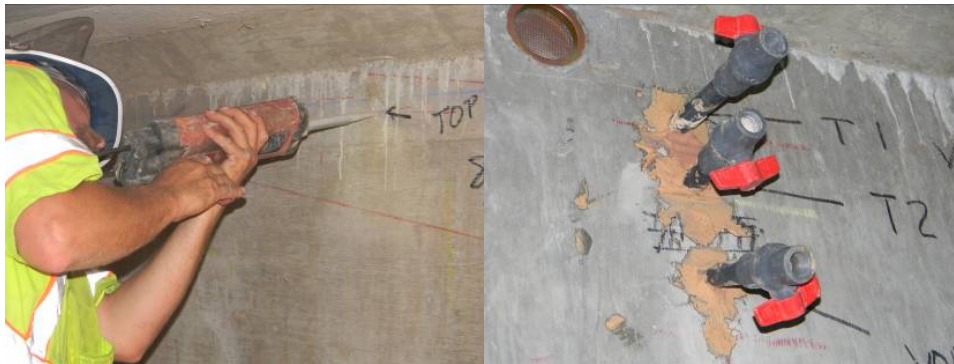
Figure 3.4. (Left) Re-sealed exposed duct holes
