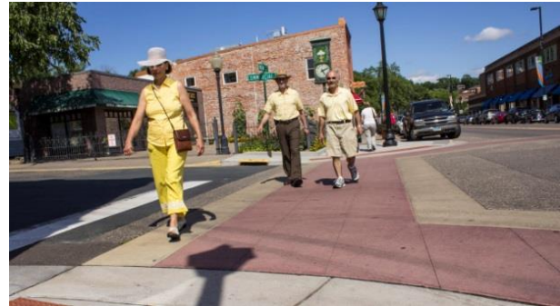
Crosswalk panels in Stillwater, MN
