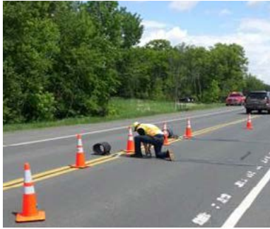
Portable weigh-in-motion systems provide a low-cost method for obtaining vehicle load distribution data.
