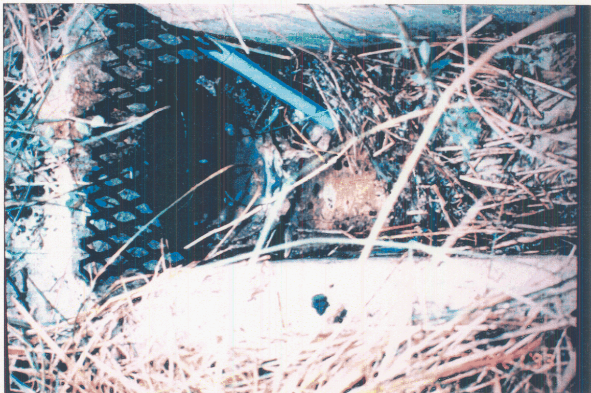
Figure 6. Rodent guard corrosion on I-90 (Austin, MN), 1994.
