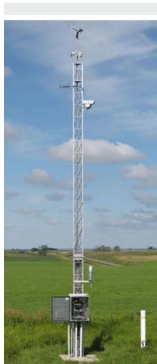
Environmental Sensor Station
