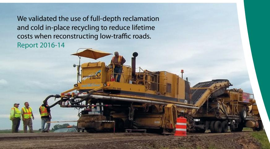
We validated the use of full-depth reclamation and cold in-place recycling to reduce lifetime costs when reconstructing low-traffic roads.
