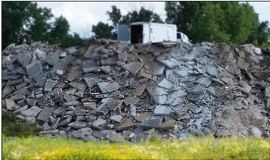
Figure 9. Concrete pavement and sidewalk for recycling.
