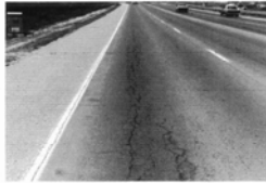
MEDIUM SEVERITY ALLIGATOR CRACKING
