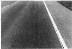
LOW SEVERITY ALLIGATOR CRACKING
