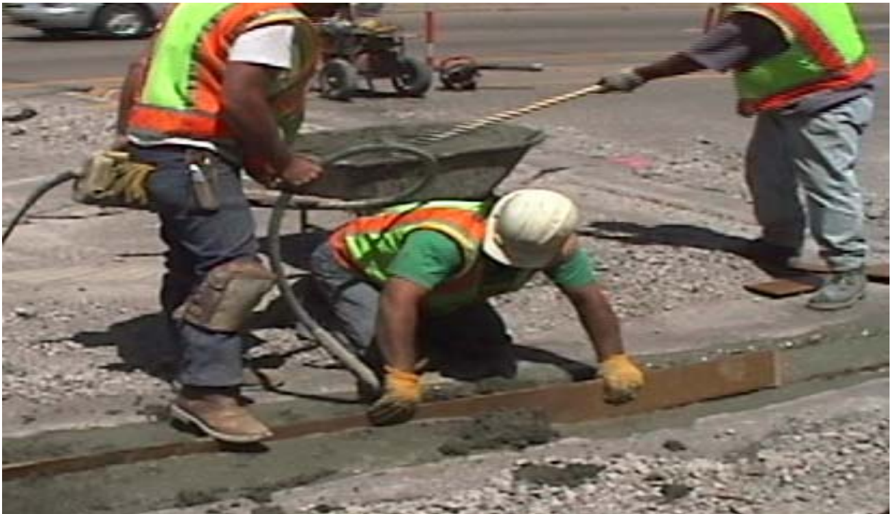
Figure 4.5 Placement of Grade 3U18 patch material and compressible insert.
