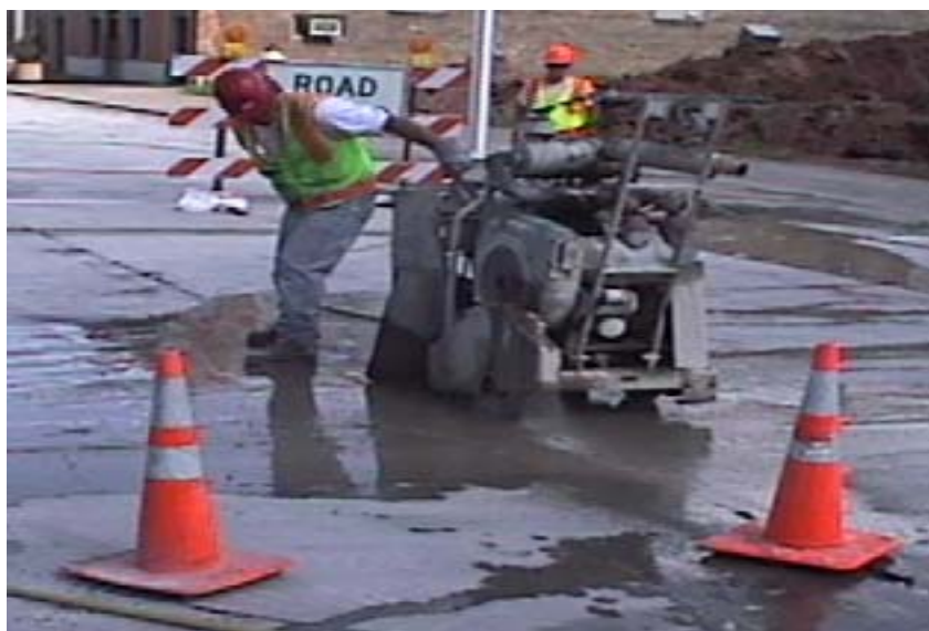
Figure 3.1 Sawing of joint before re-sealing.
