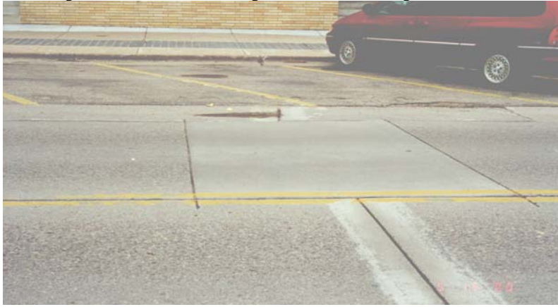
Figure 5.2 View of completed full depth repair over utility.
