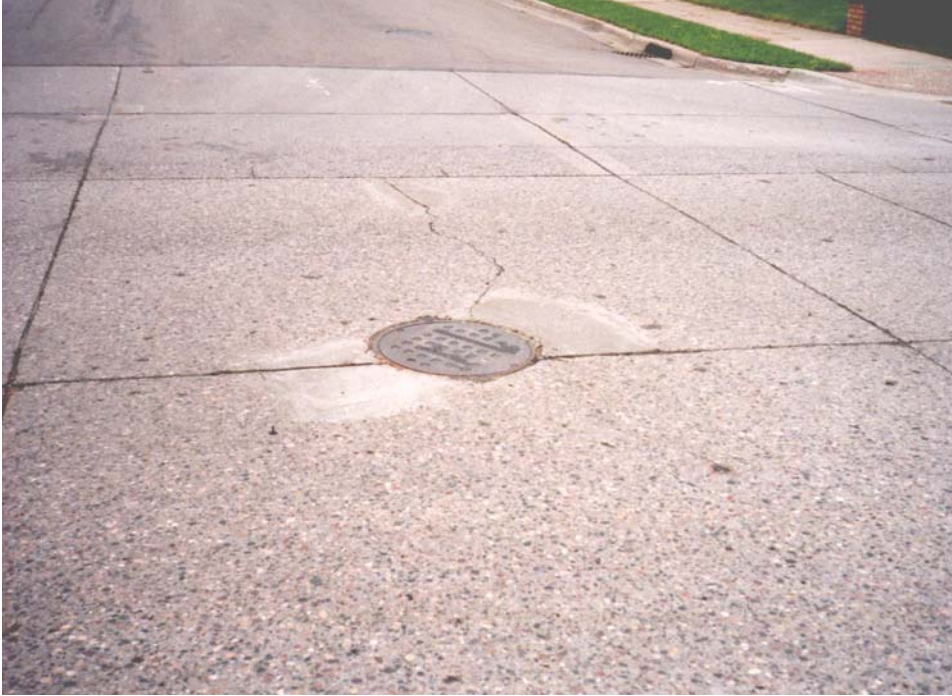
Figure 10.1 View of completed diamond ground section over manhole.
