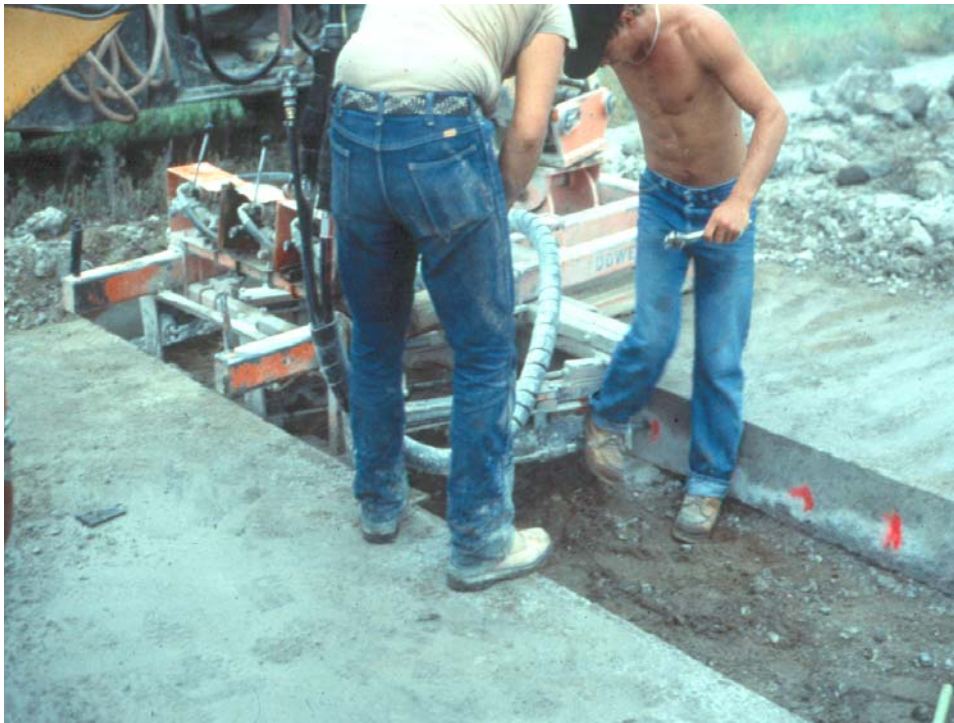
Figure 5.1 View of gang mounted drills for placement of dowels.
